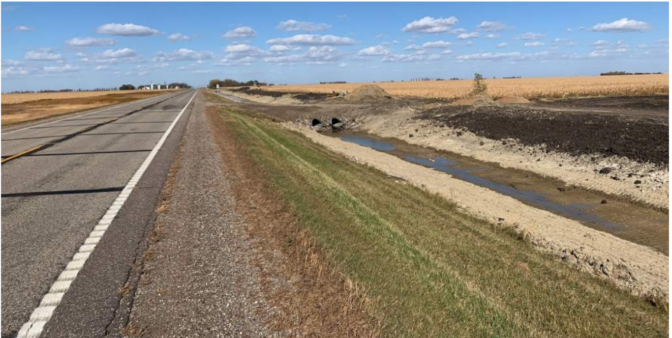
Figure 6: NS Main Section 17 – New Culverts on Field Approach (looking North)
