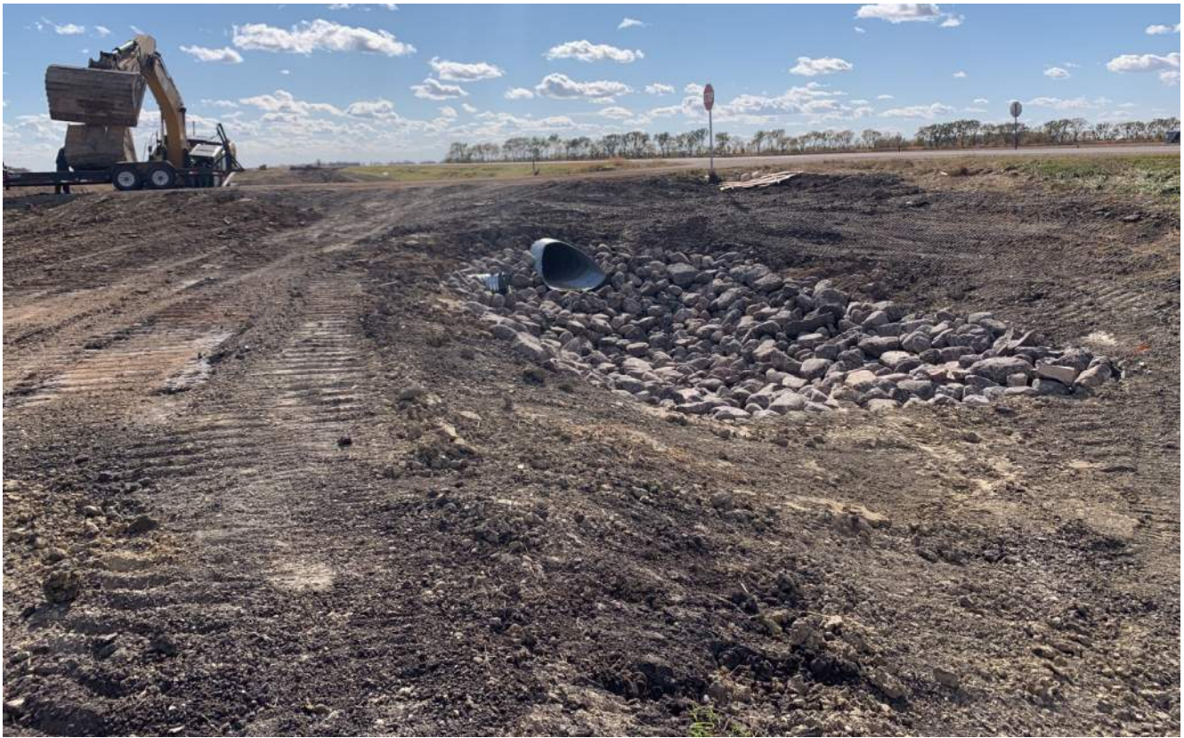
Figure 7: NS Main Section 17-20 – New Culvert on 770 th St (looking North)
