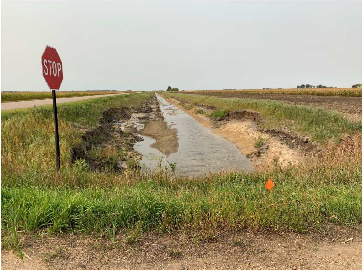
Figure 1: Erosion Area before grading 9/15/20
