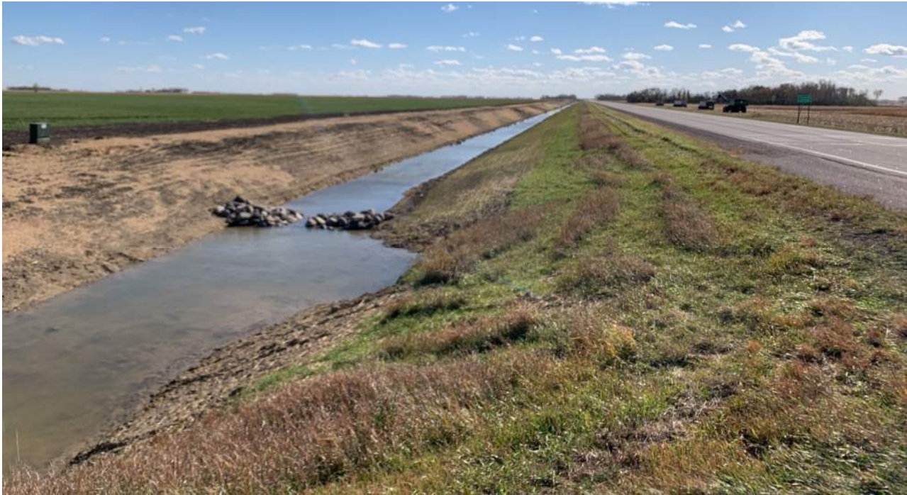
Figure 1: NS Main Section 5 (Looking South)
