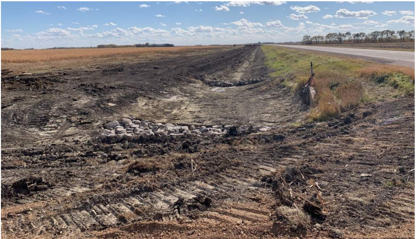
Figure 8: NS Main Section 20 (Looking South)
