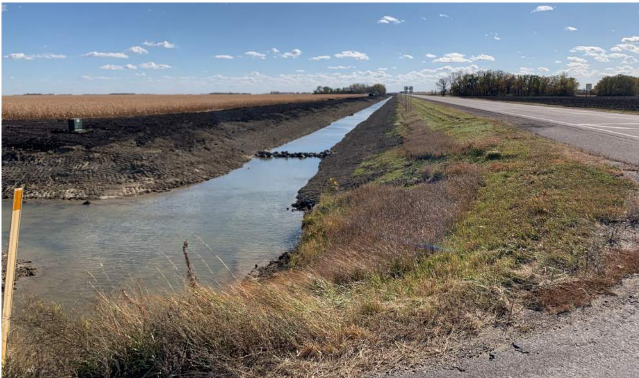
Figure 2: NS Main Section 8 (Looking South)
