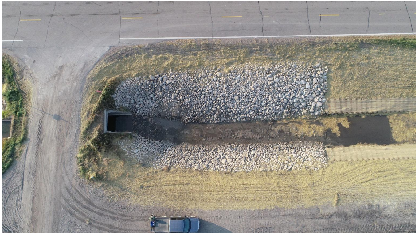
Figure 1: Erosion Area after grading and riprap. 10/9/20
