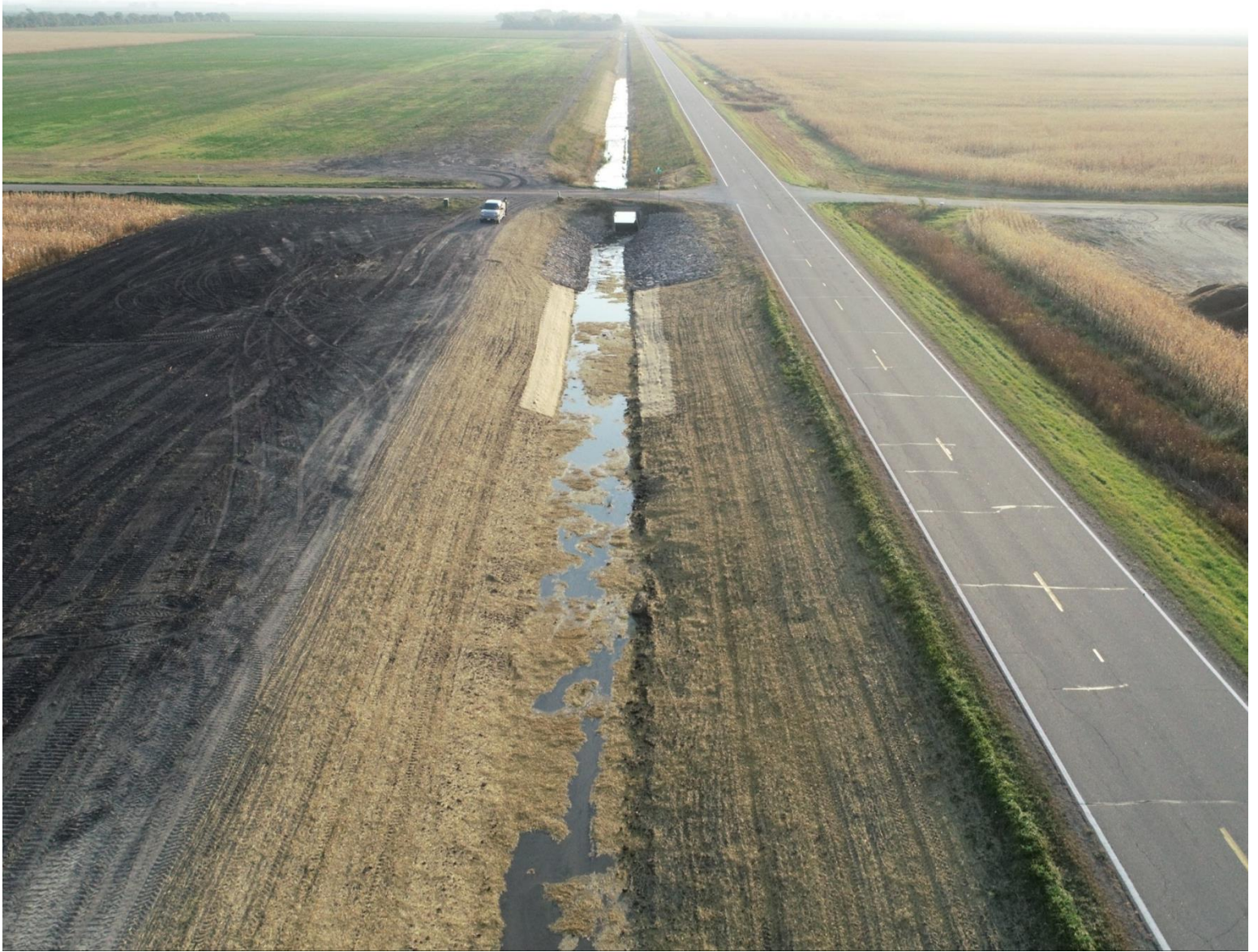
Figure 3: Looking East at previous erosion area 10/9/20
