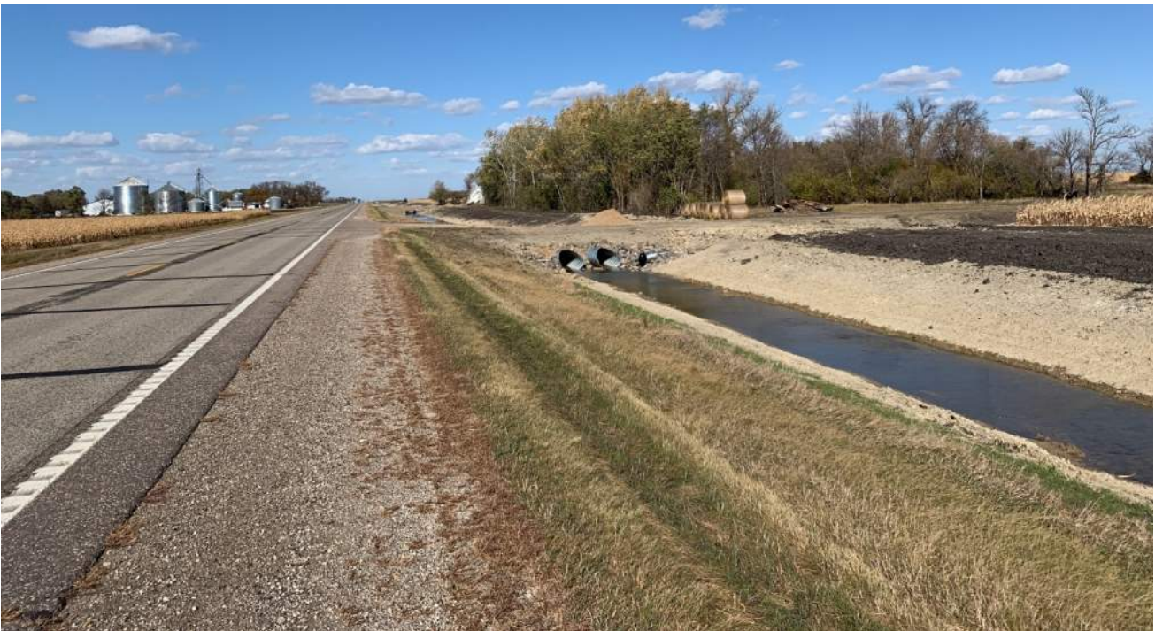
Figure 4: NS Main Section 8 – New Culverts on Field Approach (looking North)
