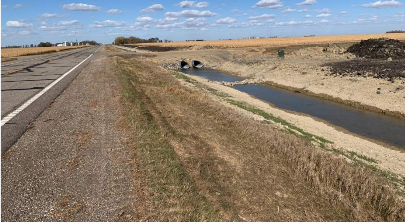
Figure 5: NS Main Section 8-17 – New Culverts on 780 th St (looking North)
